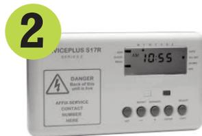
The **timer** (sometimes called a 'programmer') controls when the central heating goes on and off.
